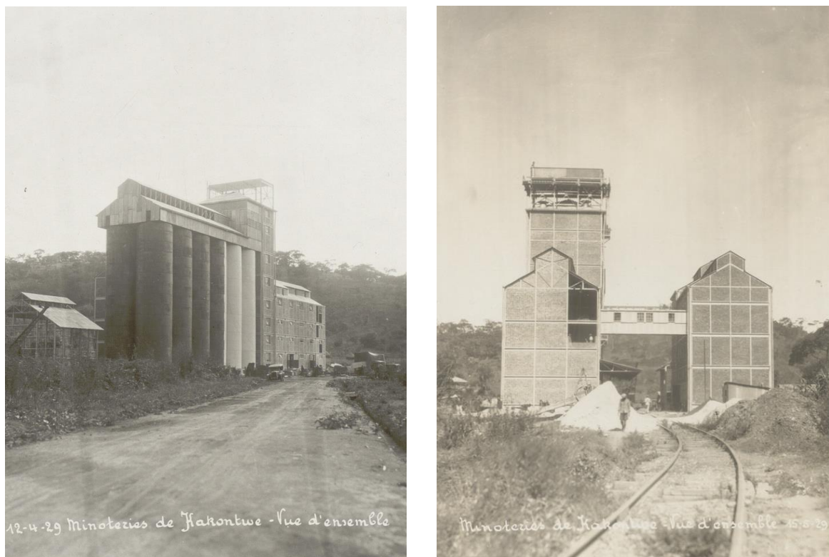
Figure 4.2 Different sides of the Kakontwe maize mill supplying the copper mines, 1929
